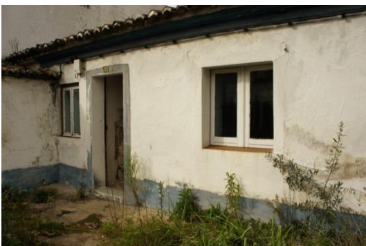
Figure 6. Monitored facade (South facade).
